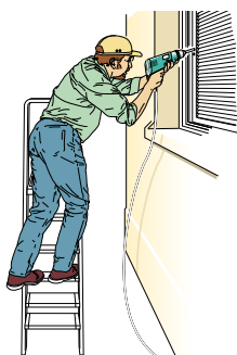
Figure 2a Incorrect - steps side-on to work activity
