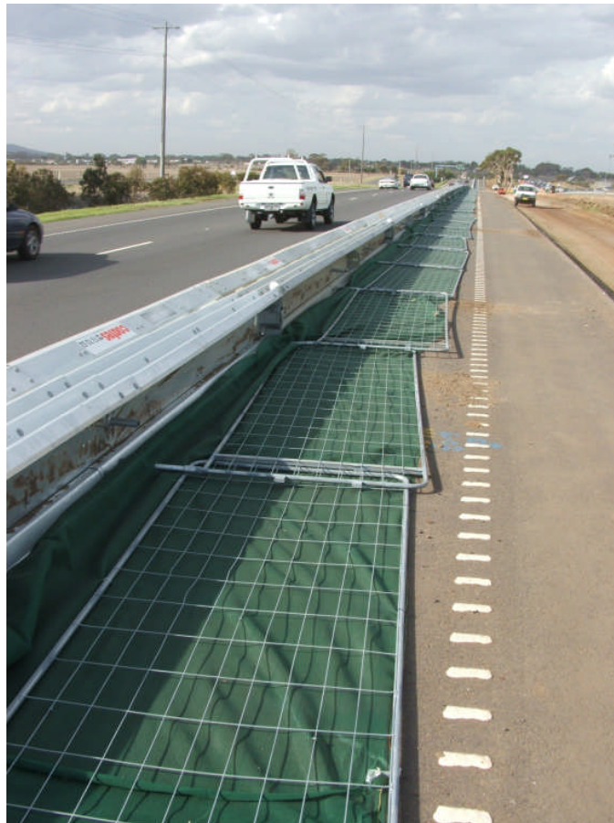
View of barriers and screens after the incident with added shade cloth
